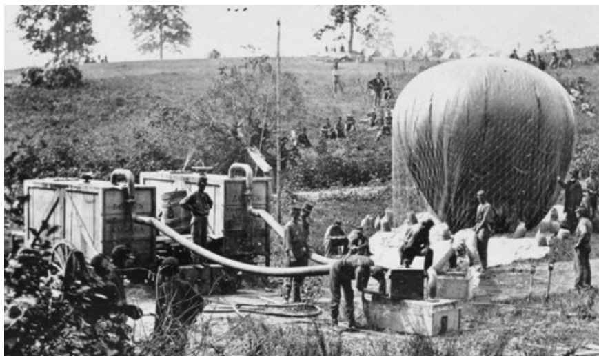
Inflating a Civil War balloon using portable hydrogen-generating equipment.
