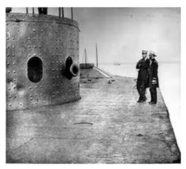
less than two feet, sufficient for coastal requirements, though a real problem when the ship went to sea. Engine power was modest, but again sufficient to the need, and a Navy requirement for masts and sails was quite appropriately ignored. The most stunning innovation, on a ship whose design was dominated by innovations, was the method of carrying her guns: a thickly-armored round turret, twenty-feet in diameter, rotated by steam power to permit nearly all-
